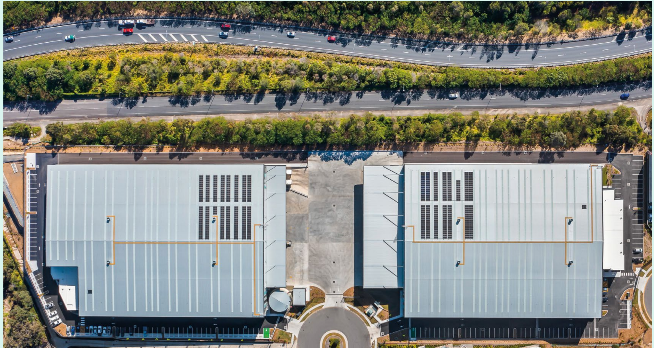
Figure 2: 100 Metroplex Place, Wacol, QLD – GPT's logistics developments include solar arrays to assist in reducing tenants' emissions.
