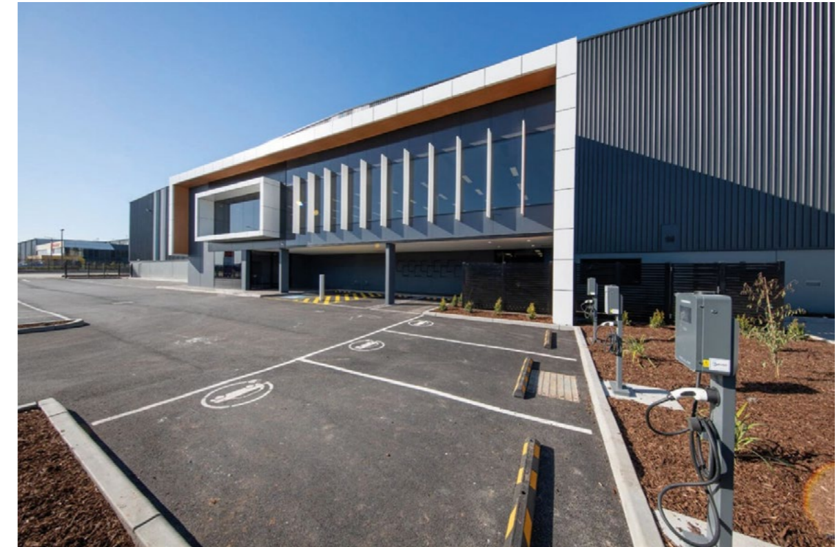
Figure 5: GPT supports the effort to lower emissions by installing EV charging stations as seen here at 143 Foundation Road, Truganina, VIC
